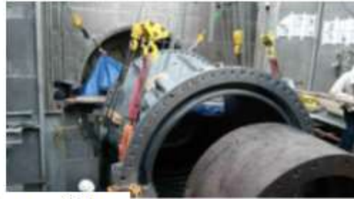
Installation of Mid Compressor Casing
