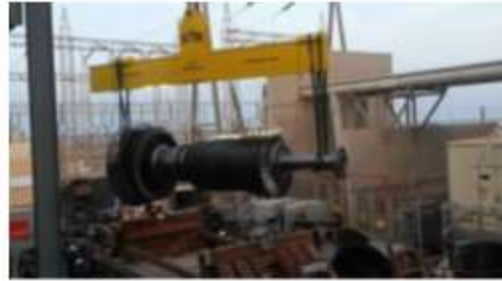
Rigging of new rotor
