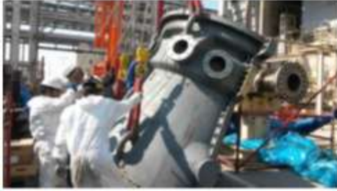
Installation of Mid Compressor Casing
